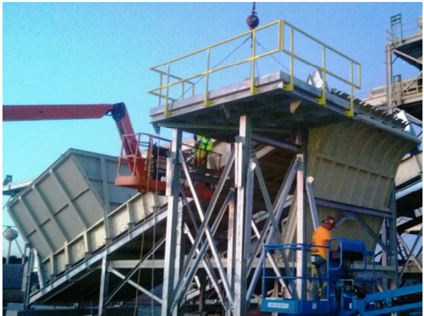
Hoppers and Structure
